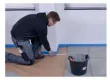
Measure the required cutouts in the room and cut individually to size. In the process, observe the necessary offset.
