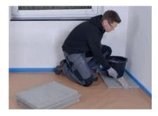
Apply the epoxy adhesive along the joint edge using a trowel and firmly press the next element against it. Min. joint width: 2 mm.
