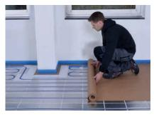
Lay a suitable pressure-resistant dry construction floor heating and roll out an overlapping separating layer (film) onto it.
