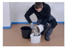
Add component B (2 kg) into component A (4 kg) and mix completely. Wear protective glasses and gloves.
