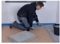
Begin with the remainder piece (≥ 20 cm) of the previous row and lay the elements with an offset (≥ 20 cm), avoiding cross joints.
