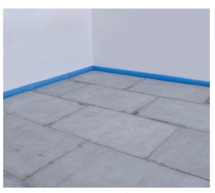
The CompactFloor EXPERT 20 is accessible and coverable after a 24-hour drying period. (Notice our material releases → Datasheets floor covering | adhesive).
