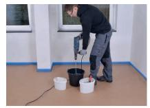
Place the mixed epoxy adhesive into a clean bucket and re-mix. The processing time for the adhesive is approx. 90 minutes (at 23°C).
