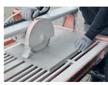
Cut the elements using a conventional diamond cutting disc without water cooling.
